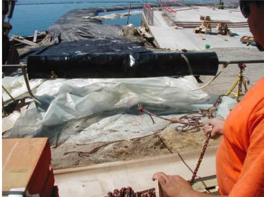
*Gently pull the string line until the rope can be grabbed. Then tie on the end of the new plastic roll and start pulling it through.*
