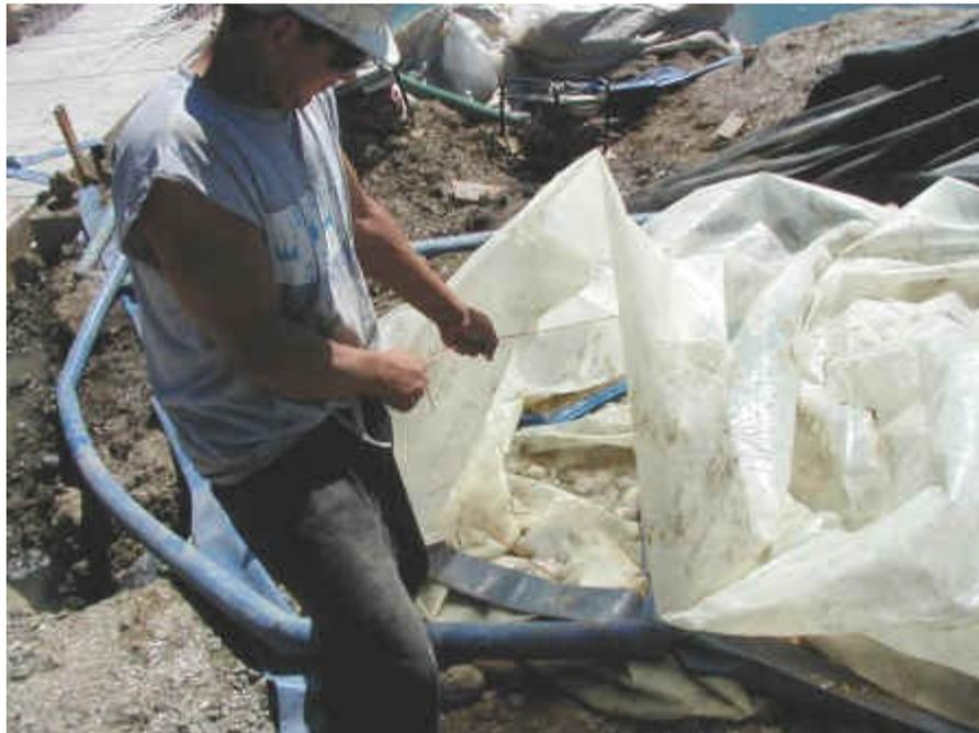
*On the far end of the AquaDam®, the roll of new inner plastic has been set up on rollers. Once the rope has been pulled through with the string line, the end of this roll will be tied onto the rope.*
