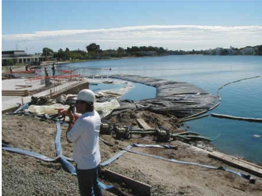
*Every large AquaDam® has string lines running through the inner tubes specifically so that they can be relined. These string lines are thin and are not for pulling the new liner through. They are simply to pull another, stronger rope through the inner tube.*
