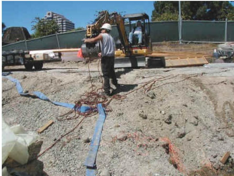
*Keep pulling until the new inner tube comes well out of the ruptured tube.*
