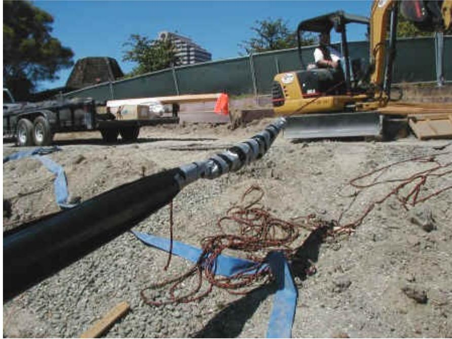
*A close-up view of the end of the new inner tube. It has been tied tightly and duct-taped in place.*
