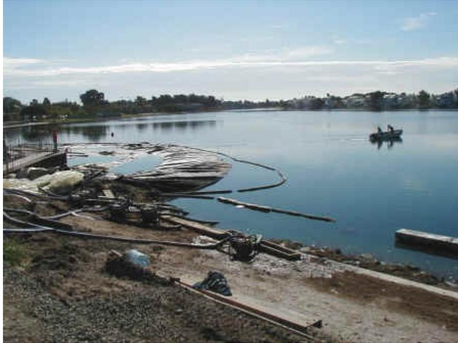
*If the AquaDam® has been moved out of position or is twisted, water must be pumped out of the AquaDam® until it is buoyant. Maneuver it until it is back in its original position. This can be done by pulling the AquaDam® manually, or, in this case, pumping water into the work area until the AquaDam® is forced out by the water pressure.*
