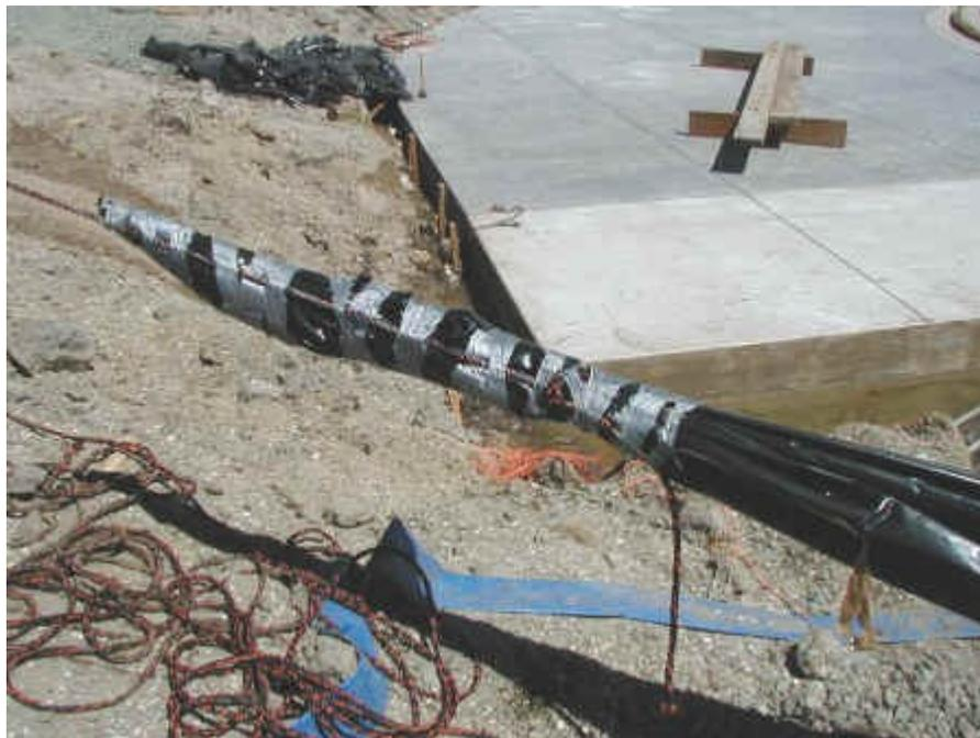
*Once the new liner is through, remove the rope and begin filling as normal.*
