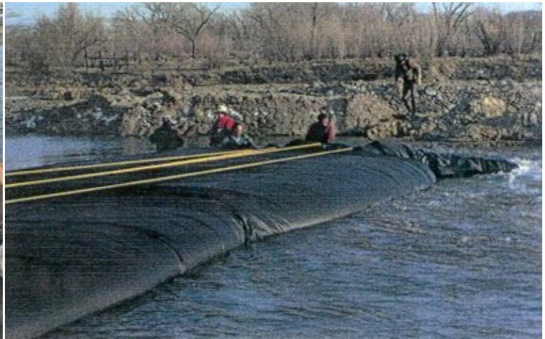
4. Unroll and fill... unroll and fill... unroll and fill... keeping continuous head inside.
