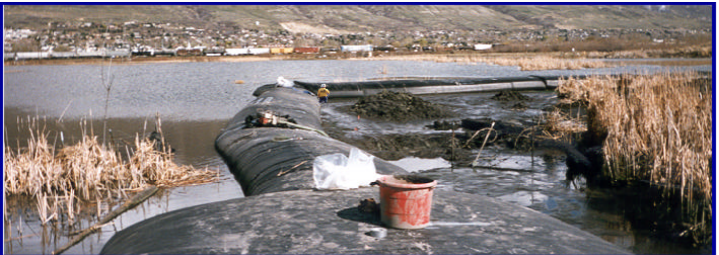
Pipeline repair at Great Salt Lake, Utah.
