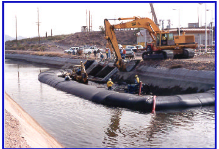
Salt River Canal Project in Phoenix, Arizona.
