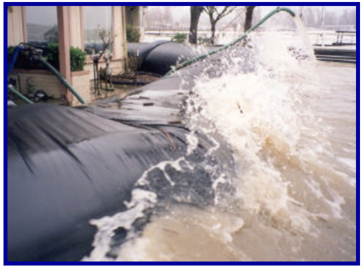
Homeowner flood control in Clear Lake, California.
