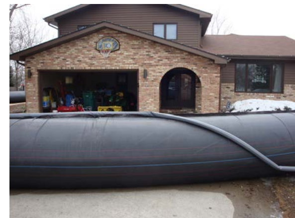
The 4' tall AquaDam is fully inflated. Elapsed time: 2 hours
