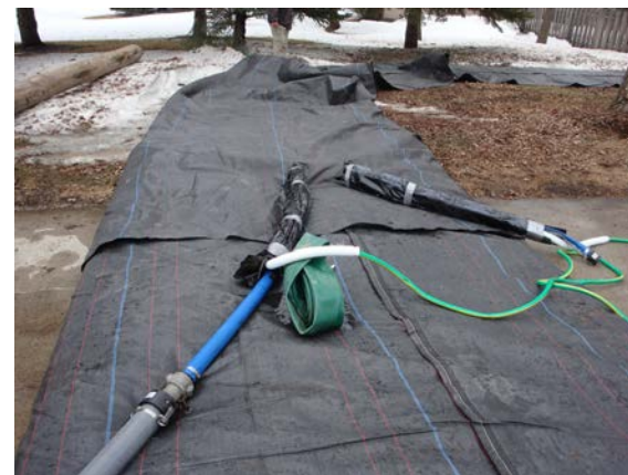
The start and end of the AquaDam use a connection collar to form a continuous floodwall
