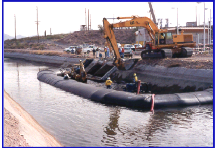
Salt River Canal Project in Phoenix, Arizona.
