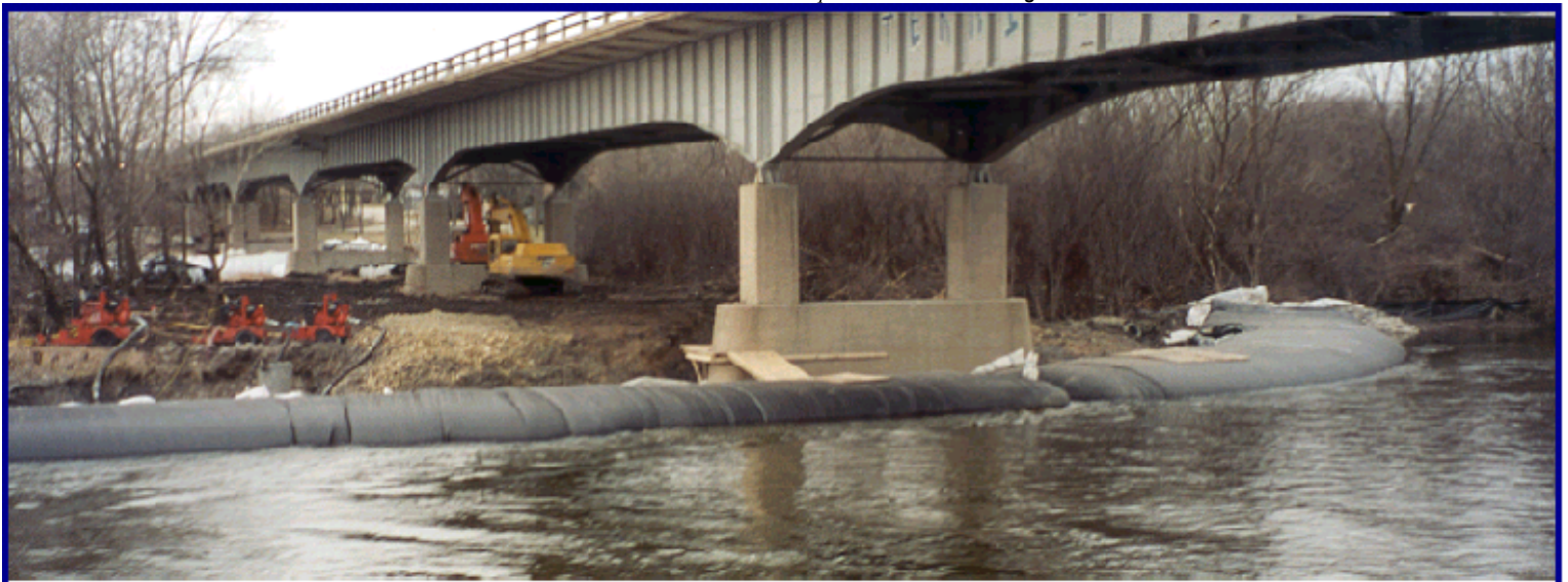
Aquadam combines weight and counter friction for an effective water-filled dam.
