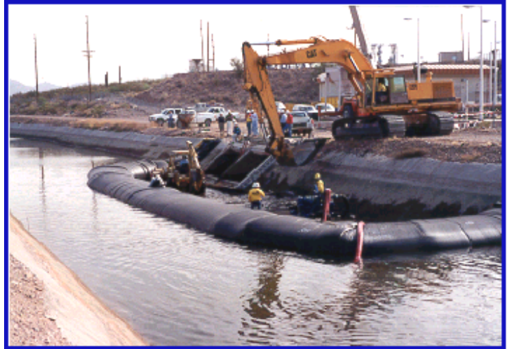
Salt River Canal Project in Phoenix, Arizona.
