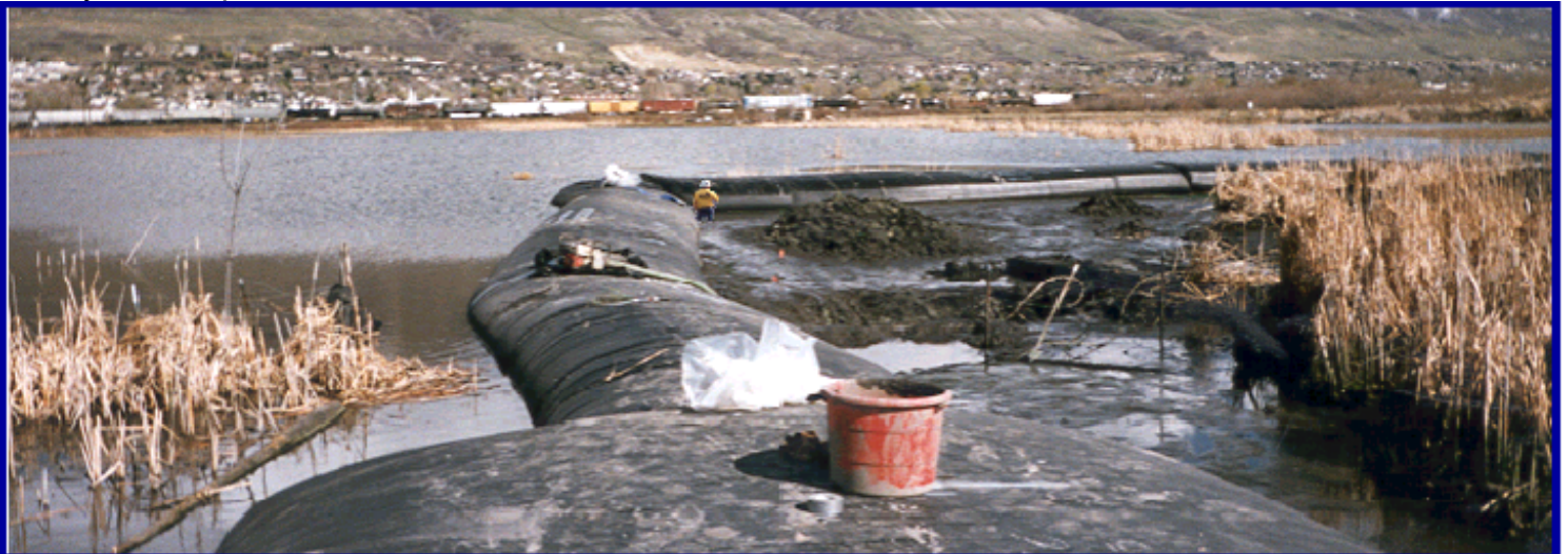
Pipeline repair at The Great Salt Lake, Utah.
